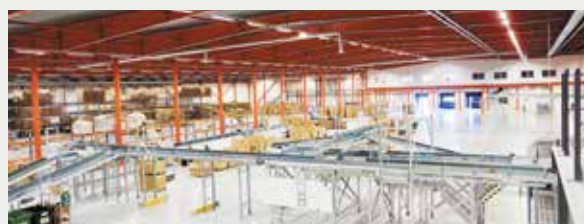
For Boozt Fashion AB Catena completed stage II of the new construction at the property Norra Varalöv 31:11 – E-City Engelholm.
