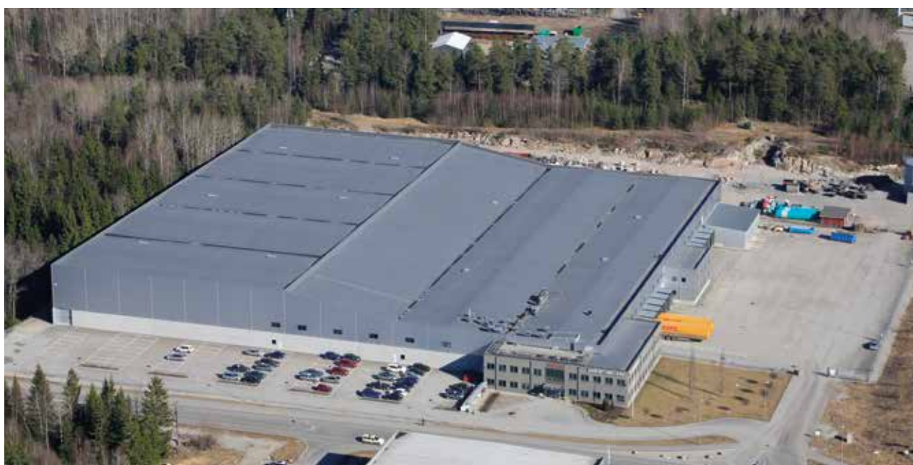
Roserberg 11:81, leased by Samdistribution. One of the properties acquired by Kilenkrysset in mid-December 2017.
