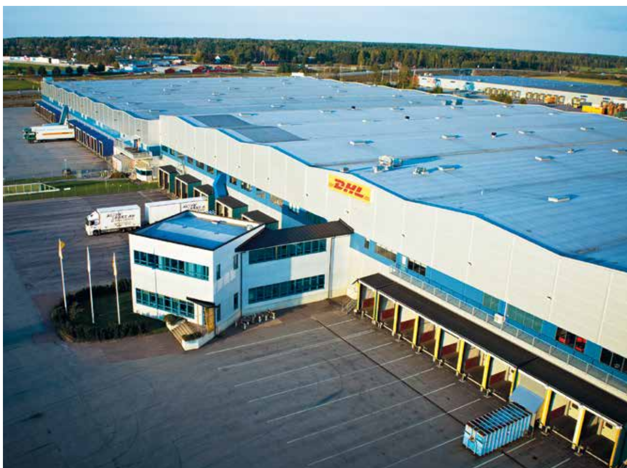
The Törsjö 2:49 logistics warehouse, located in Örebro.
