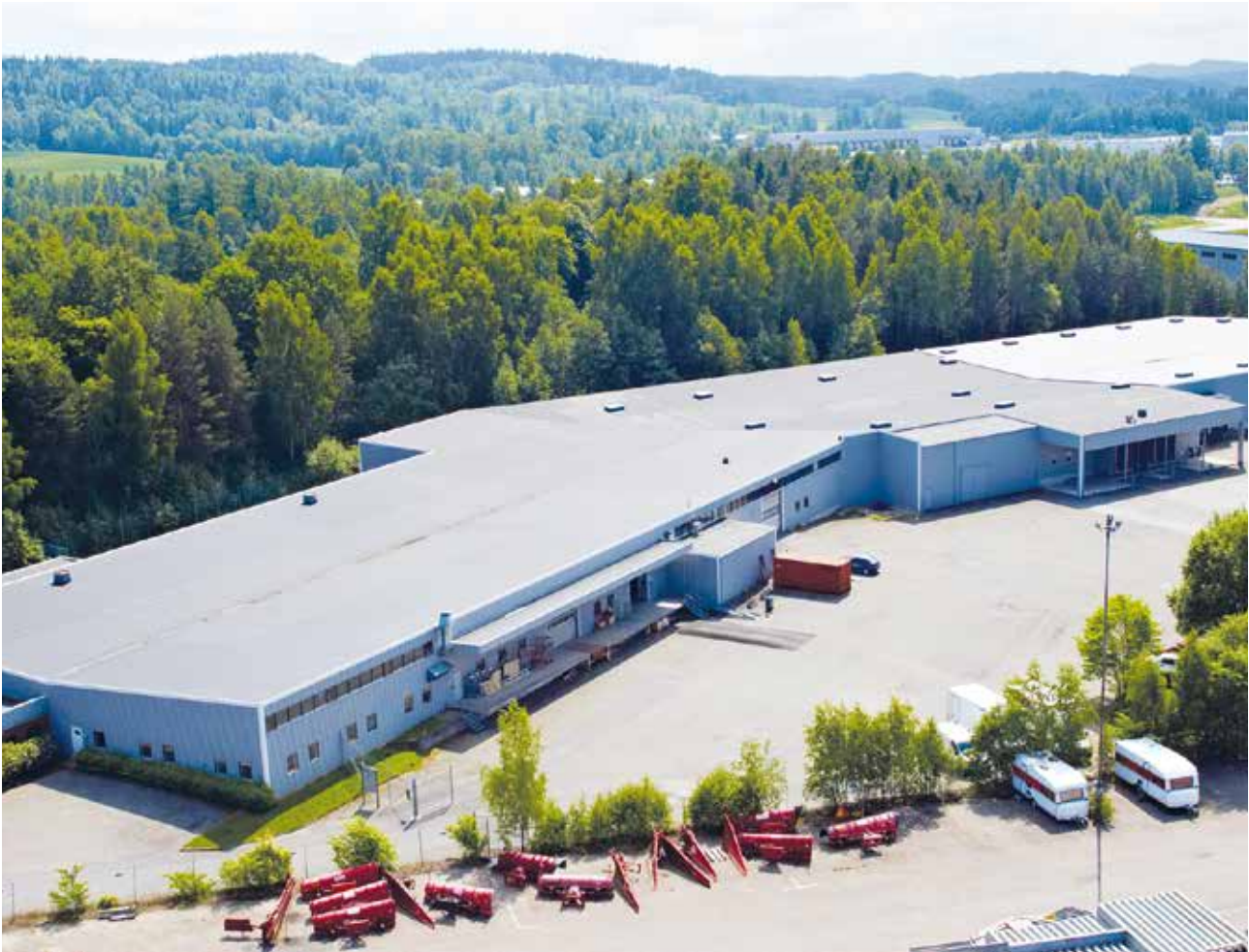
During the year, the Ättehögen 2 logistics warehouse in Jönköping was equipped with a geothermal heating system that reduces both costs and environmental impact.
